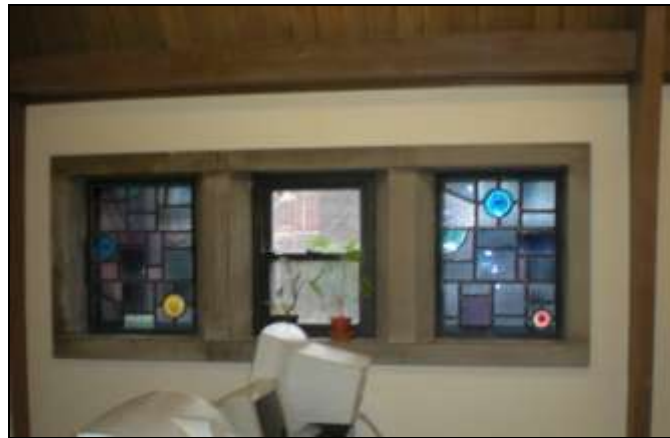
Concrete Frame around three windows.
