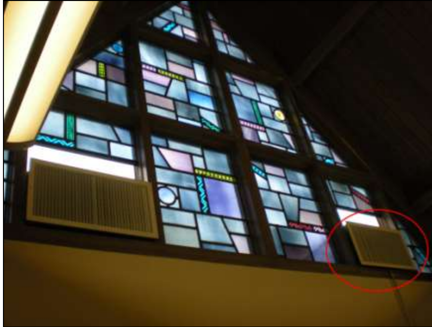
Air Exhaust Vent on North face of church.
